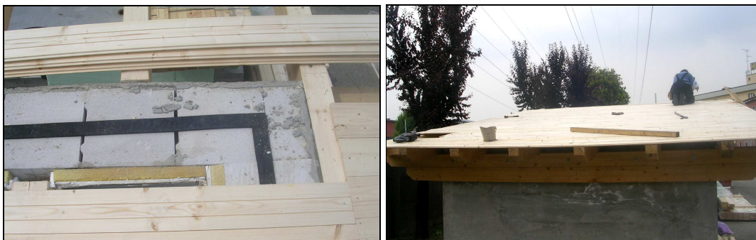
Figure 10: construction of the first wooden boarding; detail wall - roof connection
