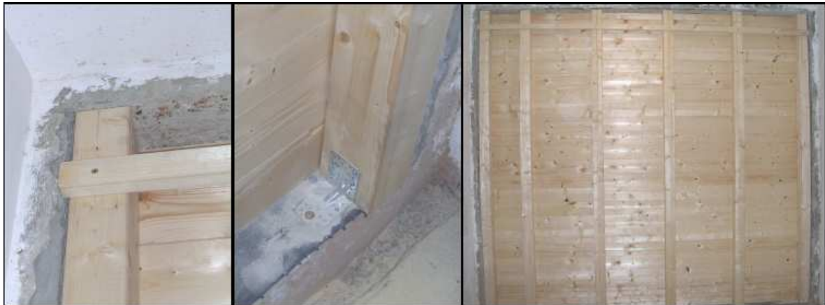
Figure 1: Receiving room side - basic wooden structure, from left to right: higher part, lower part, basic wooden structure
