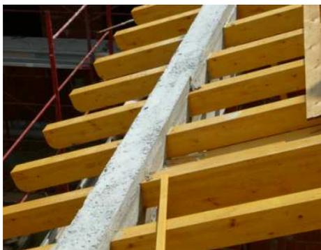
**Figure 22.** Secondary beams built passing through the edge beam
