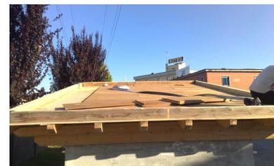
**Figure 13.** Lateral wood retaining beams
